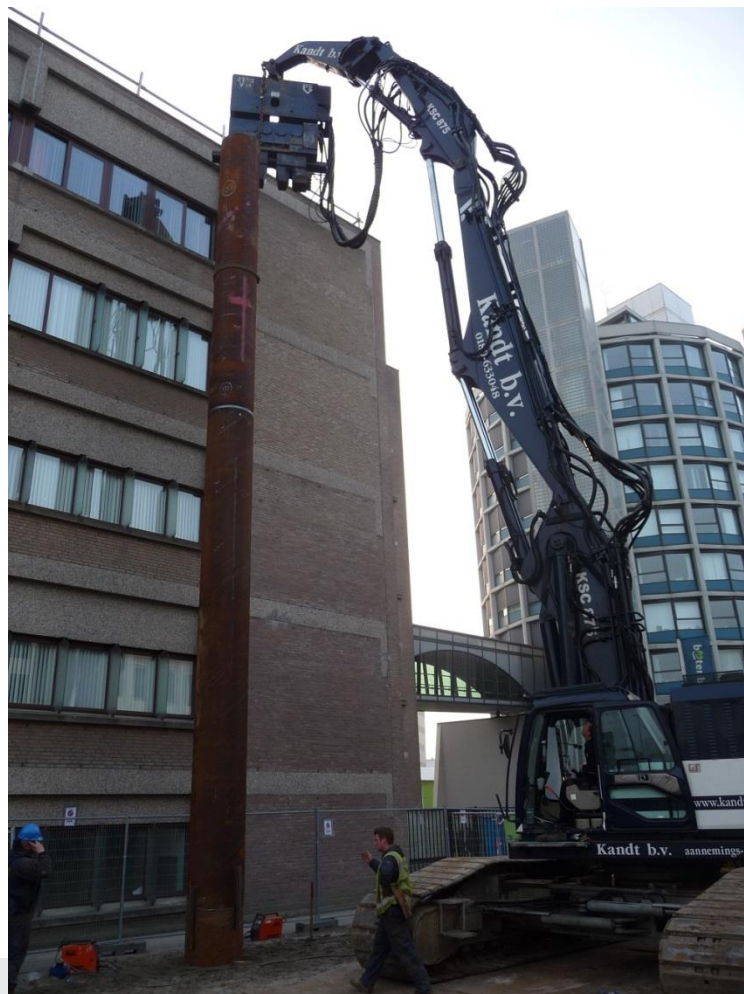
Intrillen stalen casing.
